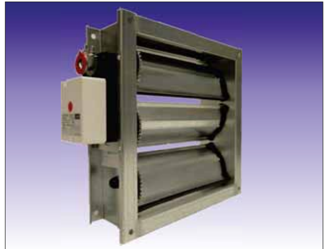
ATG DAMPER with CMR Actuator
